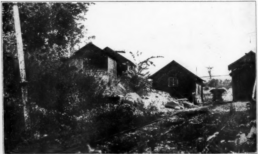
Buildings at Top of Quarry
